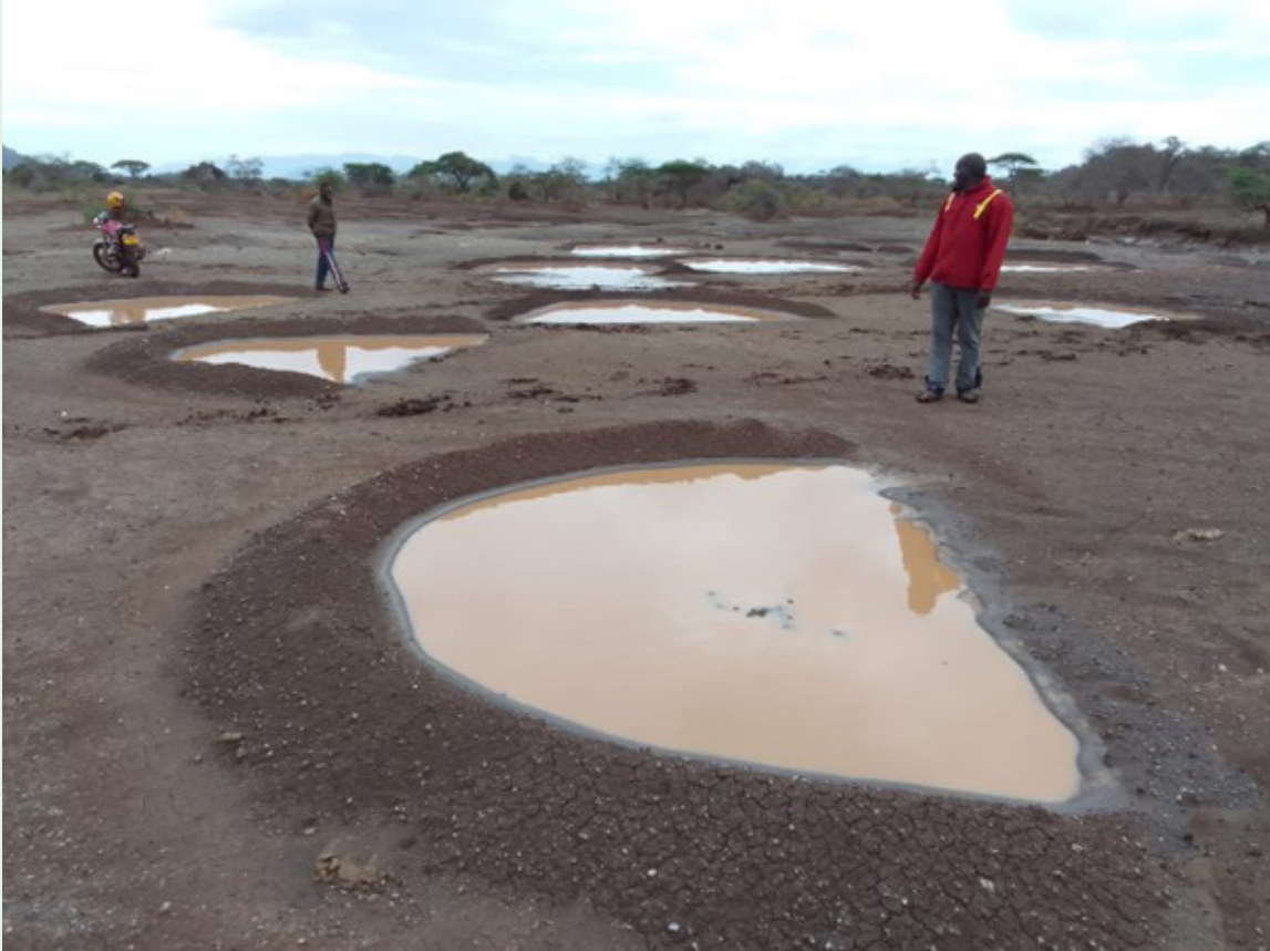
Figure 8. Bunds holding water after the rains in December 2022.
