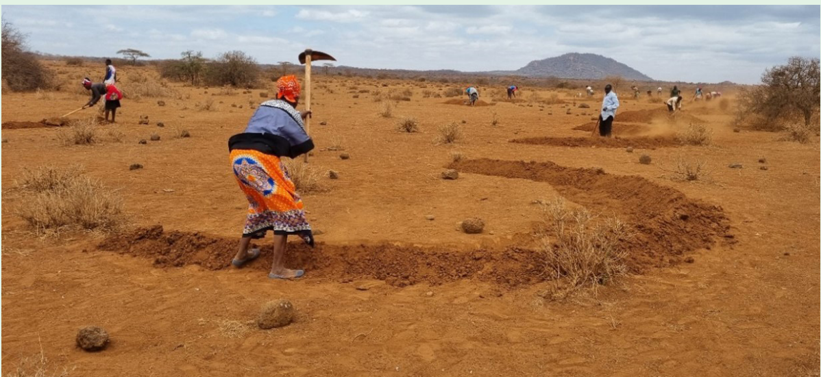
Figure 7: Ongoing bund digging.
