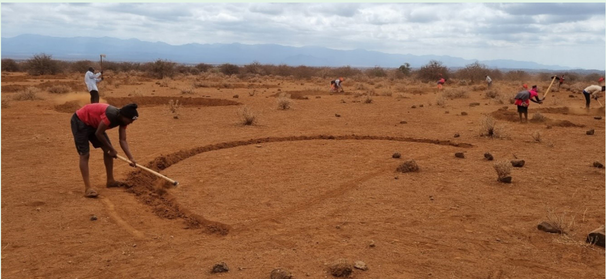
Figure 6: Digging of bunds at Rombo.
