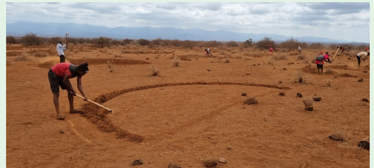
Figure 6: Digging of bunds at Rombo.
