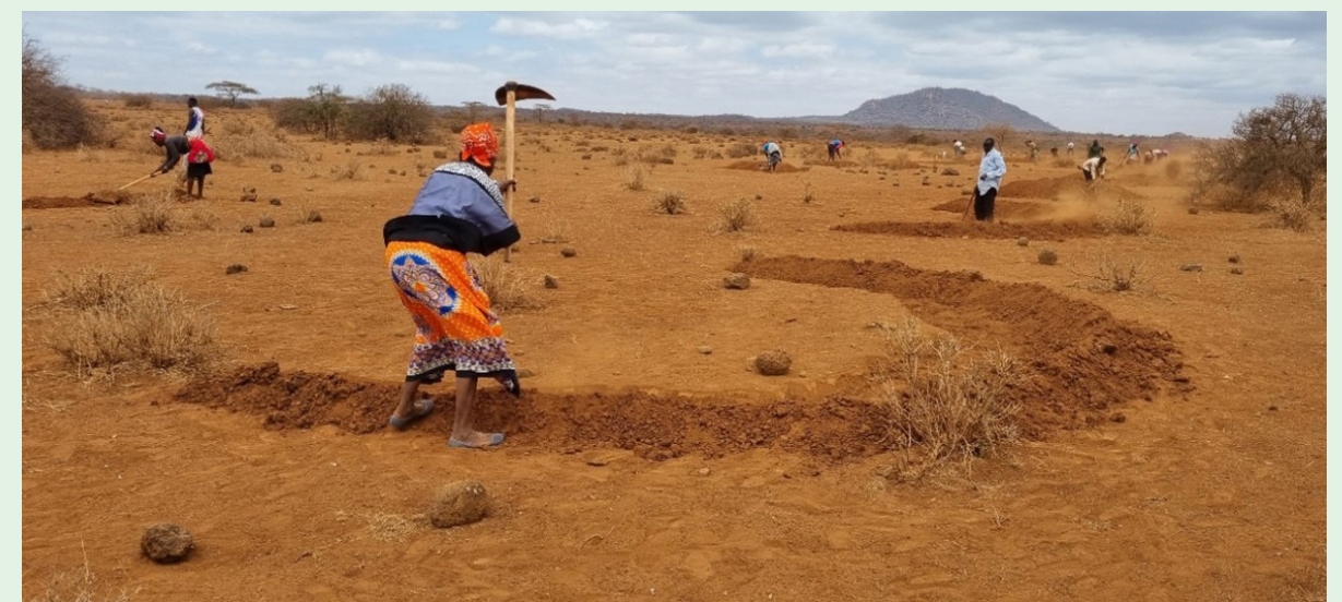
Figure 7: Ongoing bund digging.
