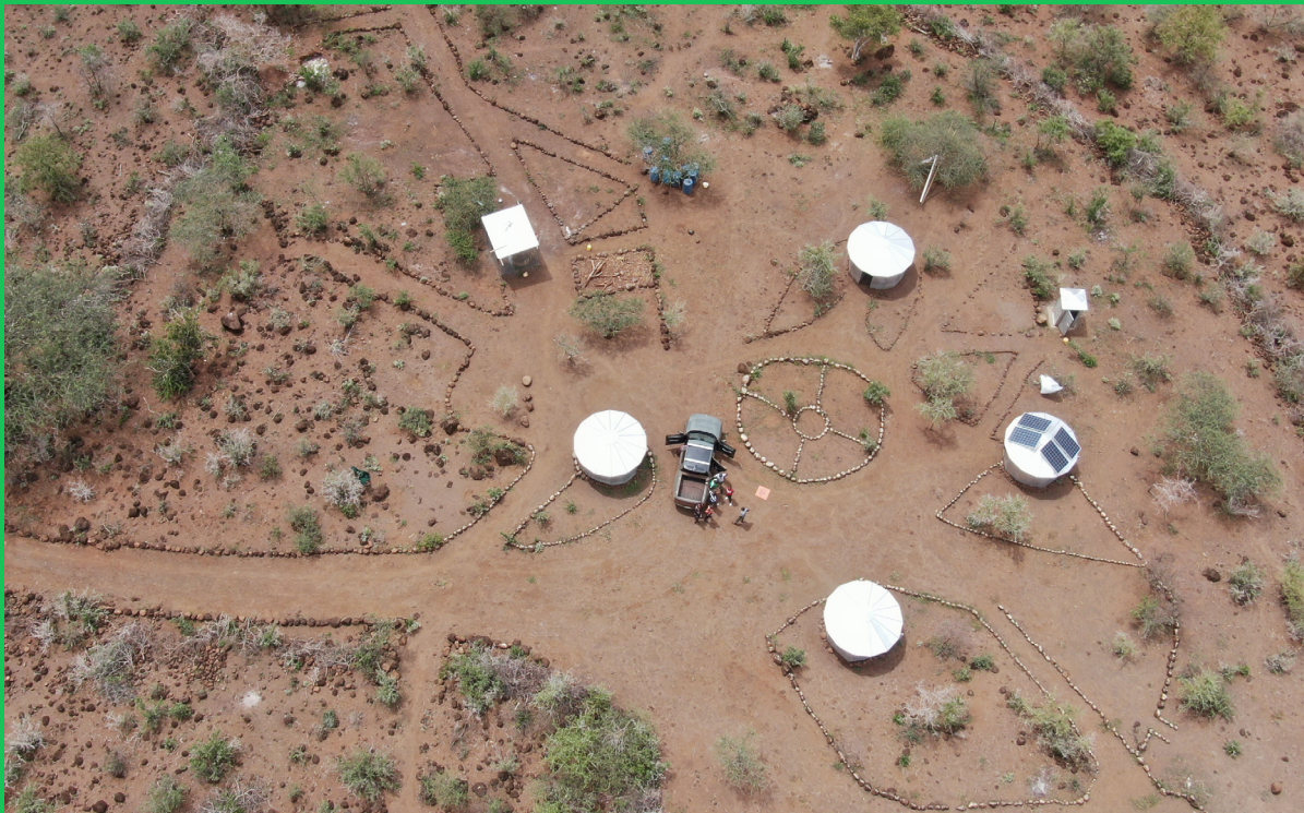
FIGURE 5: ROMBO RANGERS POST INSIDE THE BUND SITE
