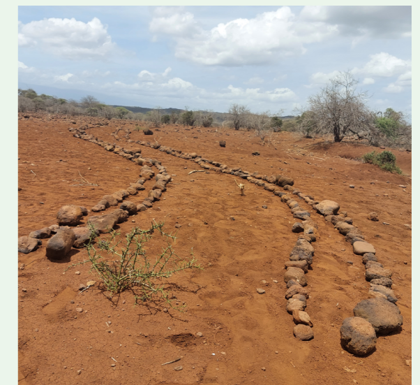
FIGURE 2 & 3: ROMBO BUNDS AND STONE LINES DURING BUND DIGGING IN JAN 2023
