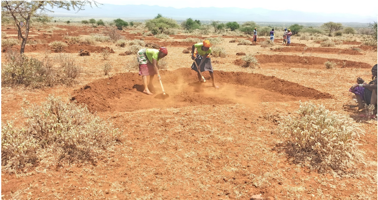
Figure 4: Bund digging in Ilchalai
