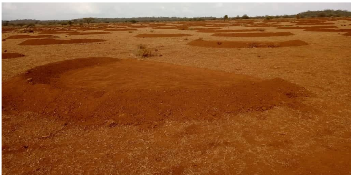
Figure 7: Bunds dug in Ilchalai
