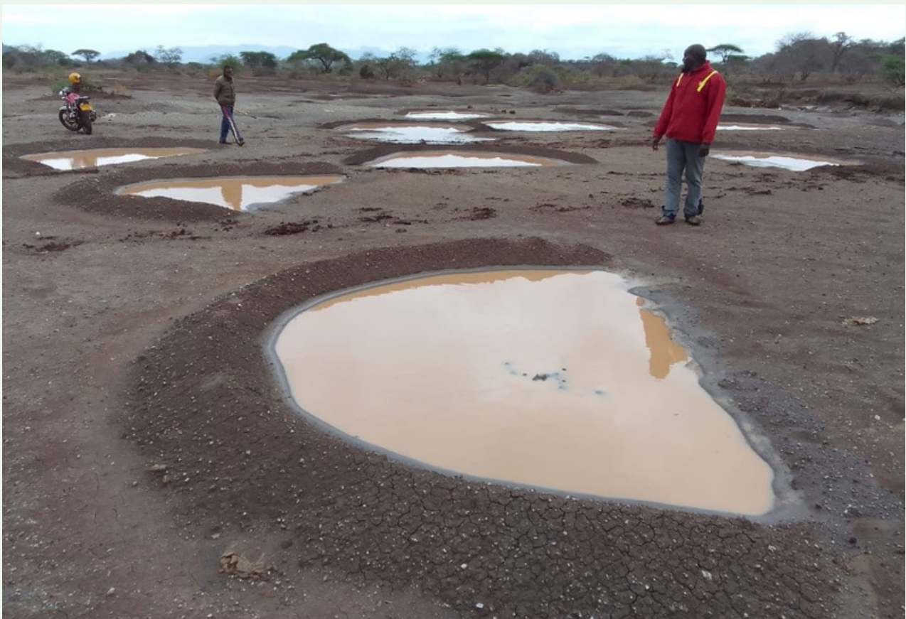
Fig 9. Bunds after the first rains. There has so far been only 1 rain shower, which is concerning, we need follow up rains but at least the bunds are holding water and that is great.
