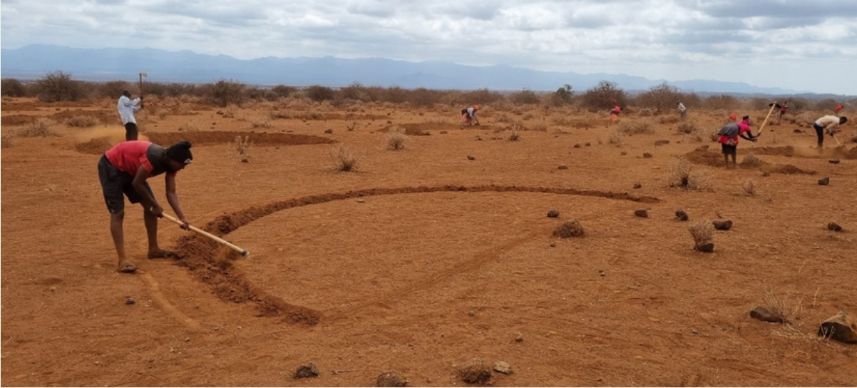
Fig 6. Digging of bunds
