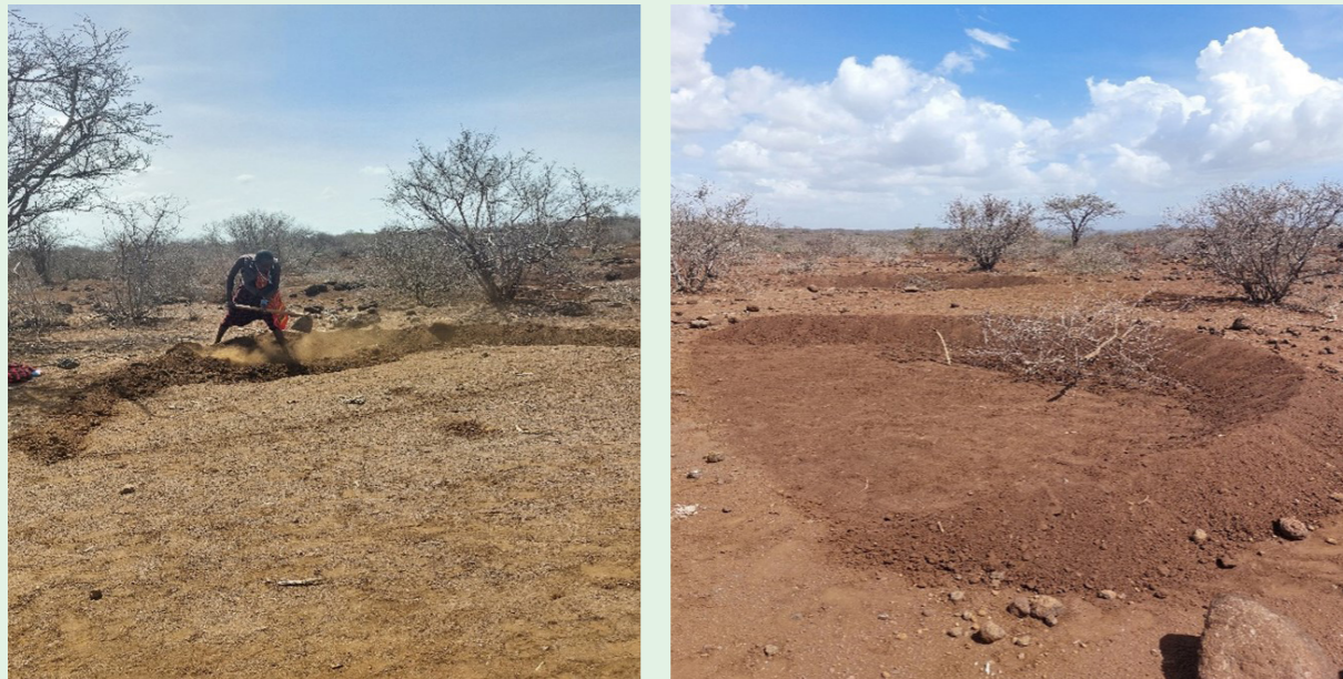
Figure 10: Rombo digging ongoing in anticipation of the March to April 2023 rains.
