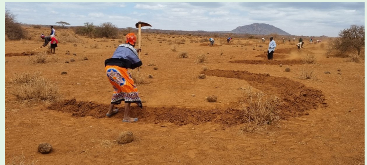
Figure 7: Ongoing bund digging.
