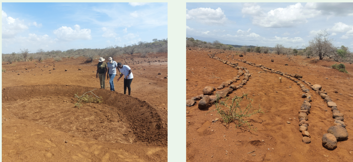
FIGURE 2 & 3: ROMBO BUNDS AND STONE LINES DURING BUND DIGGING IN JAN 2023
